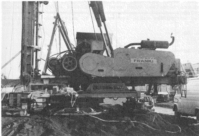
Fig. 2b Franki rig instrumentation with data acquisition system
